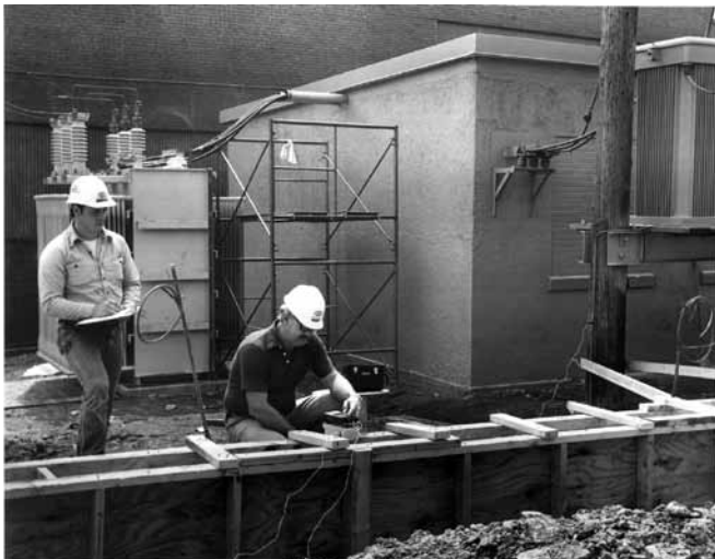
Checking the earth resistance of a ground system at a substation using a Megger ground tester, Cat. No. 250260
