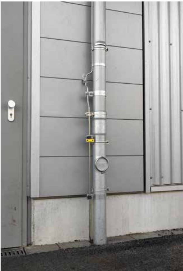
Figure 2.18: Lightning down-conductor at a downpipe
