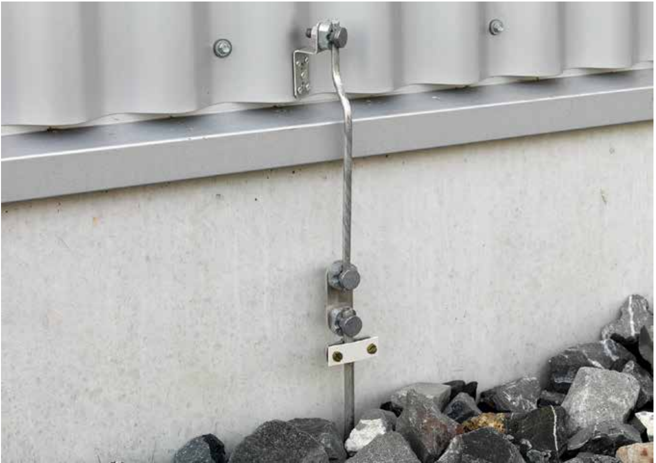
Figure 4.1: Separation point on a metal facade
