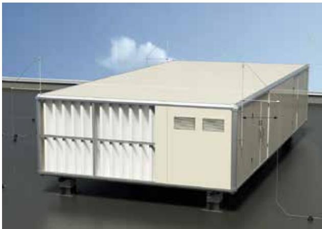
Fig. 2.28: Insulated interception system with separation distance (s)
