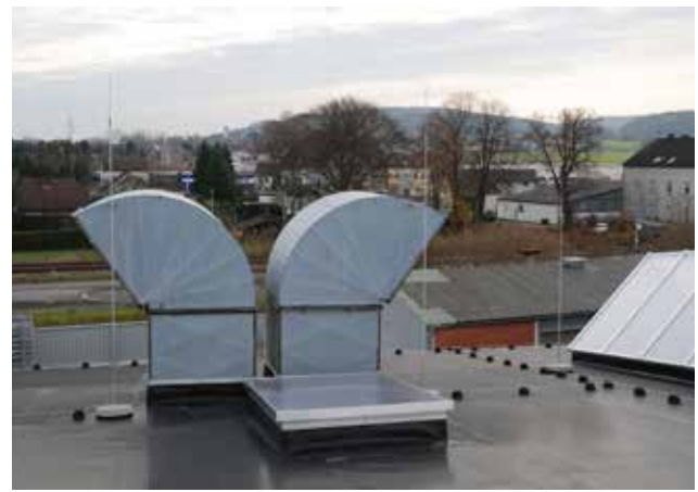
Figure 2.24: Isolated system with GRP holders
