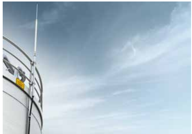
Figure 2.58: Isolated lightning protection with isCon®
