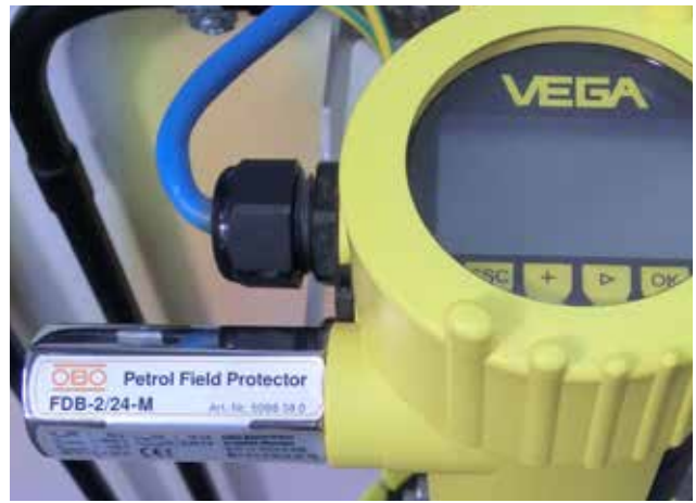
Figure 3.66: Sensor with Petrol Field Protector (see item 7 in Figure 3.68)
