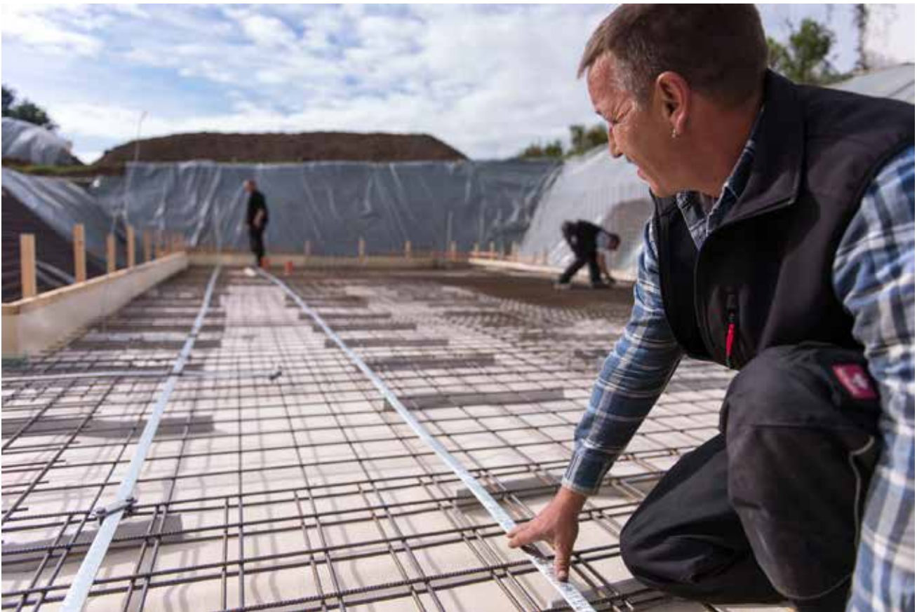
Figure 2.75: Installing a foundation earther
