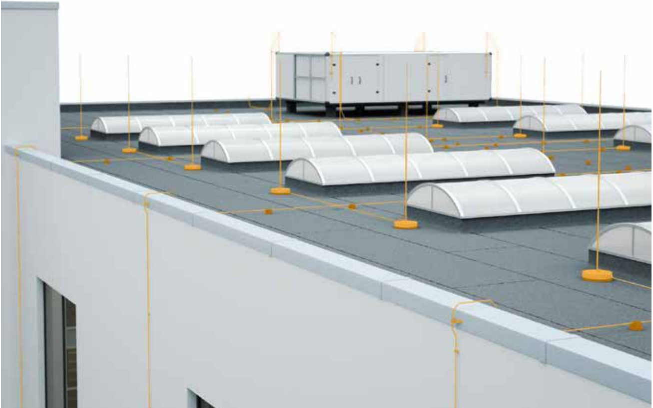
Figure 2.14: Natural components (here: metal of roof parapet) for air-termination systems, IEC 62305-3 (VDE 0185-305-3)
