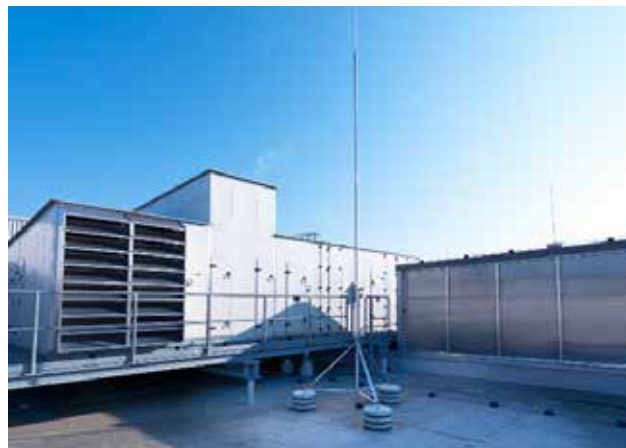
Fig. 2.29: Aluminium air-termination rod
