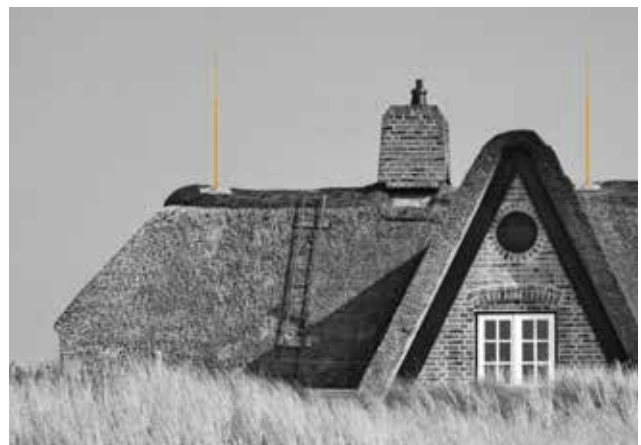
Figure 2.71: Soft-covered roof with isCon®
