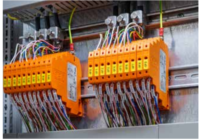
Figure 3.44: SAS clamp clip to connect the shielding braid with MDP surge protection devices
