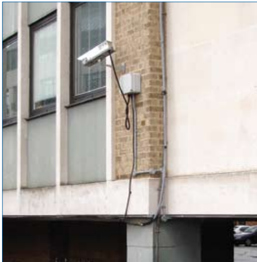
Figure 65. Conventional down-conductor separation distance problem.
