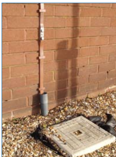
Figure 51. Typical down-conductor connectors.
