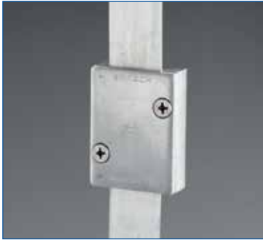
Figure 50. Typical down-conductor test joints.
