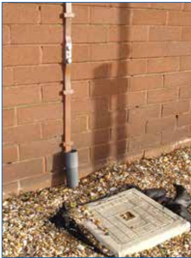
Figure 51. Typical down-conductor connectors.
