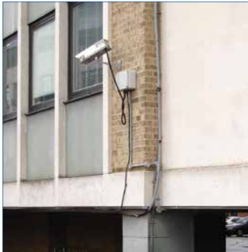
Figure 65. Conventional down-conductor separation distance problem.
